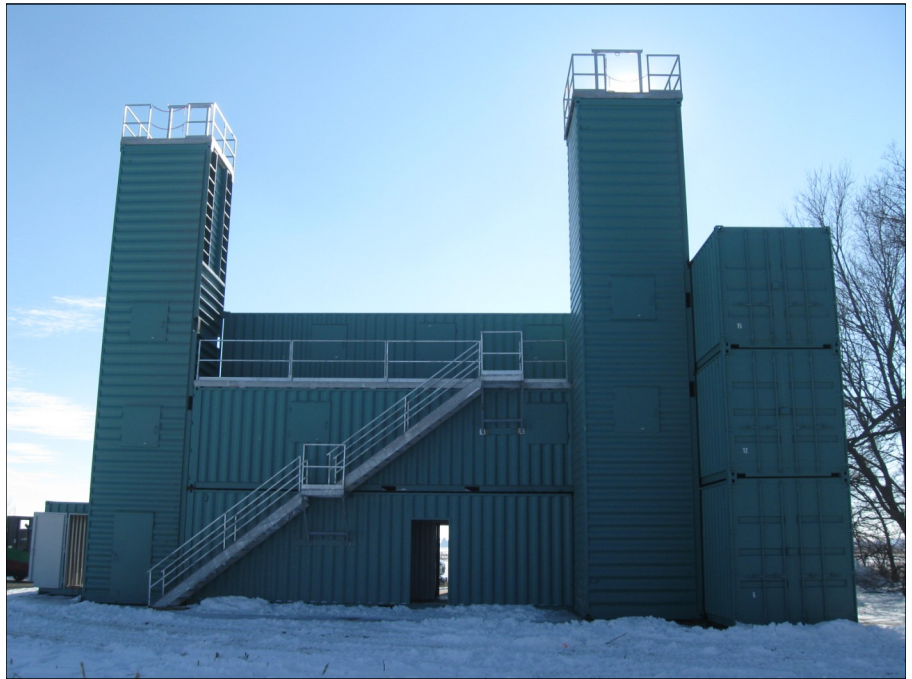
Live Fire Training Facility purchased with $200,000 grant from the Illinois Department of Commerce and Economic Opportunity
